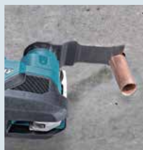
Flush copper pipe cutting
