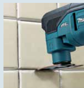
Tile grout removal
