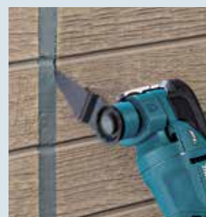
Elastic sealant removal
