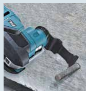
Flush rebar cutting
