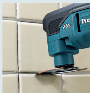
Tile grout removal
