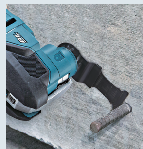
Flush rebar cutting
