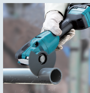
PVC pipe cutting
