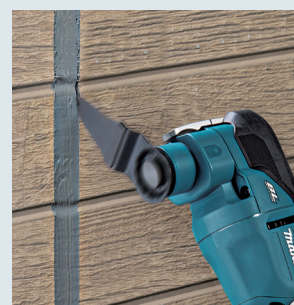
Elastic sealant removal
