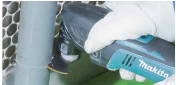
Cutting PVC, FRP pipes
