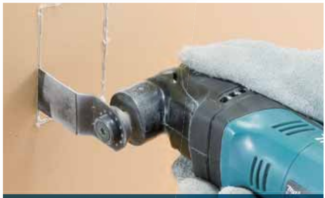
Cutting plasterboards
