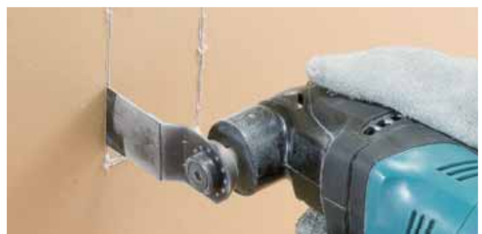
Cutting plasterboards
