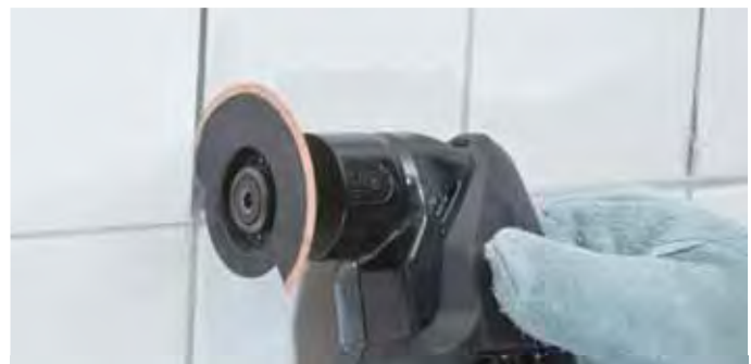
Routing joints on wall tiles
