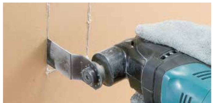
Cutting plasterboards
