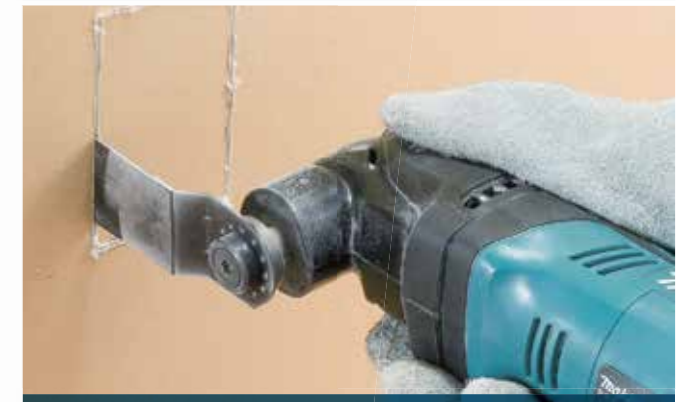
Cutting plasterboards
